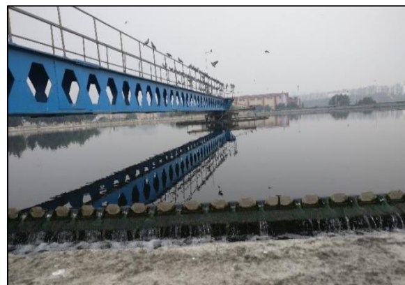
Fig 7: Secondary Clarifier of Okhla Plant
