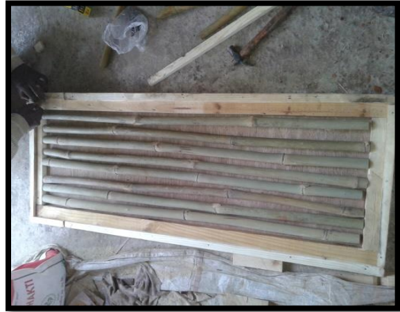
Fig 8(d): Preparation of Bamboo Panel
