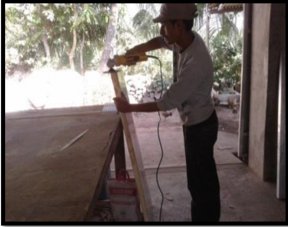
Fig 8(n): Preparation of Bamboo Panel
