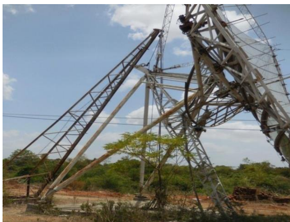
Fig 4: Crematorium Tracking stand Aligned with Back Crane and Reflector Frame
