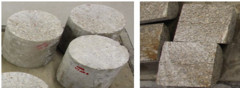
Figure 10: Surface Cracks Healed in Specimens with Large Cracks Healing under WD Cycles, and Internal Crack after Cutting the Cylinder Transversally to the Crack
